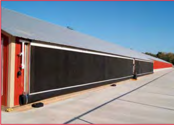
Figure 113: Example of a cooling pad.
