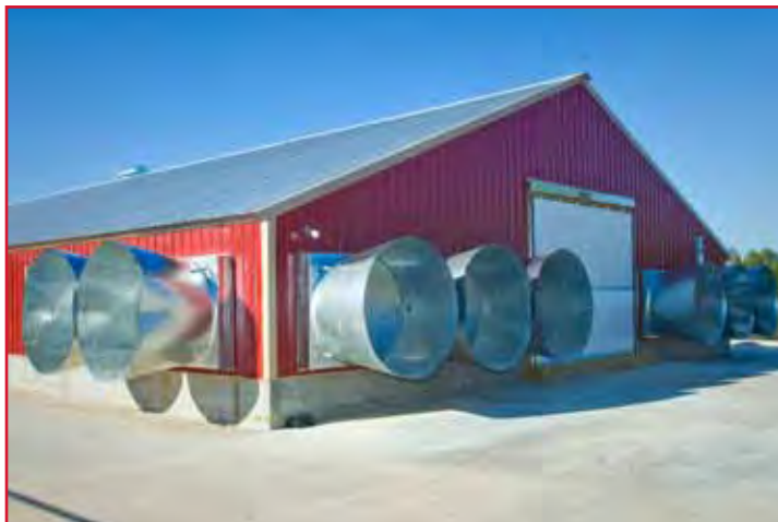
Figure 109: Example of a typical tunnel ventilated house.
